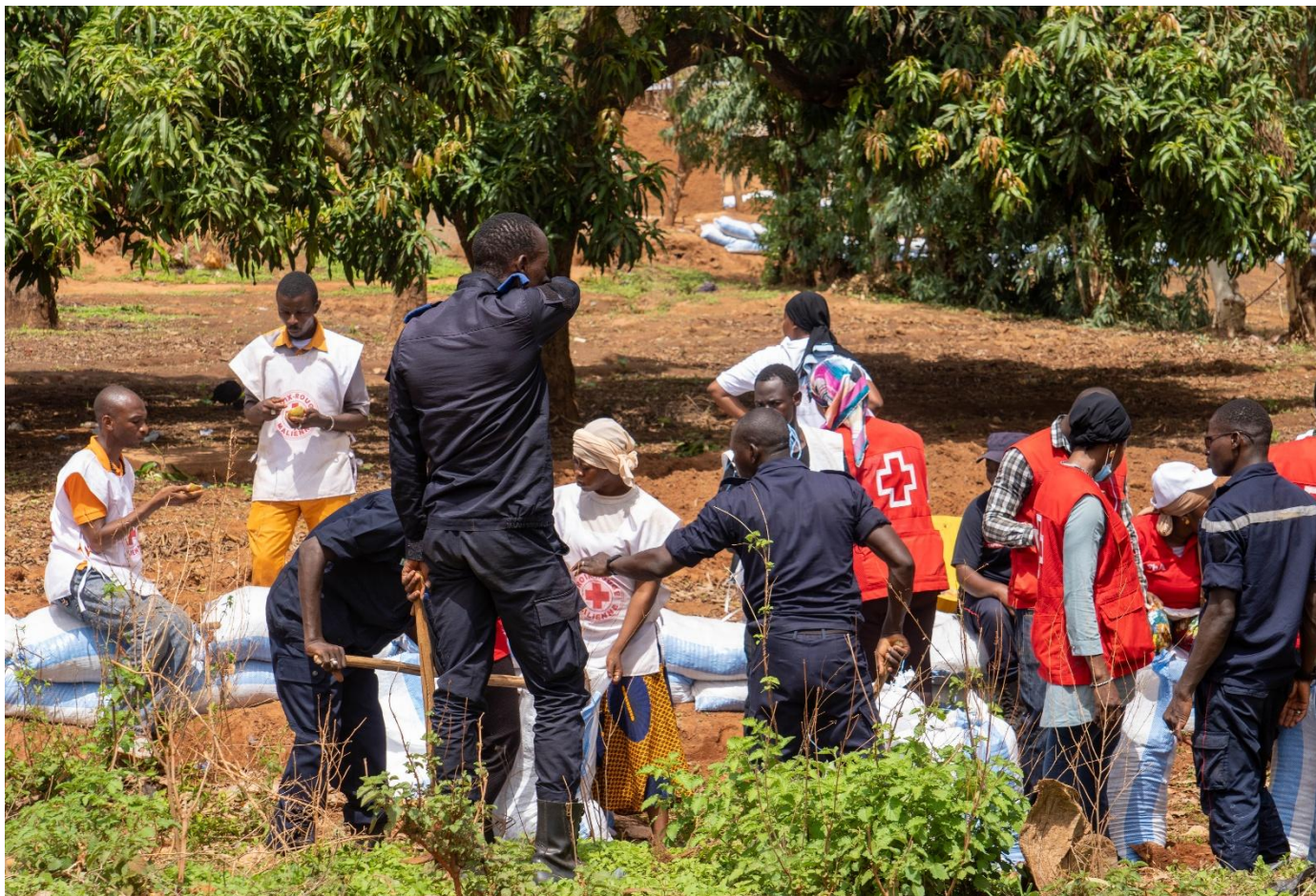
Red Cross of Mali (CRM) volunteers reinforce protective dikes using sandbags during a simulation exercise ("Dry Test") of the Early Action Protocol for riverine flooding in the Sikasso region, aimed at testing anticipatory actions and community mobilization ahead of the rainy season.
